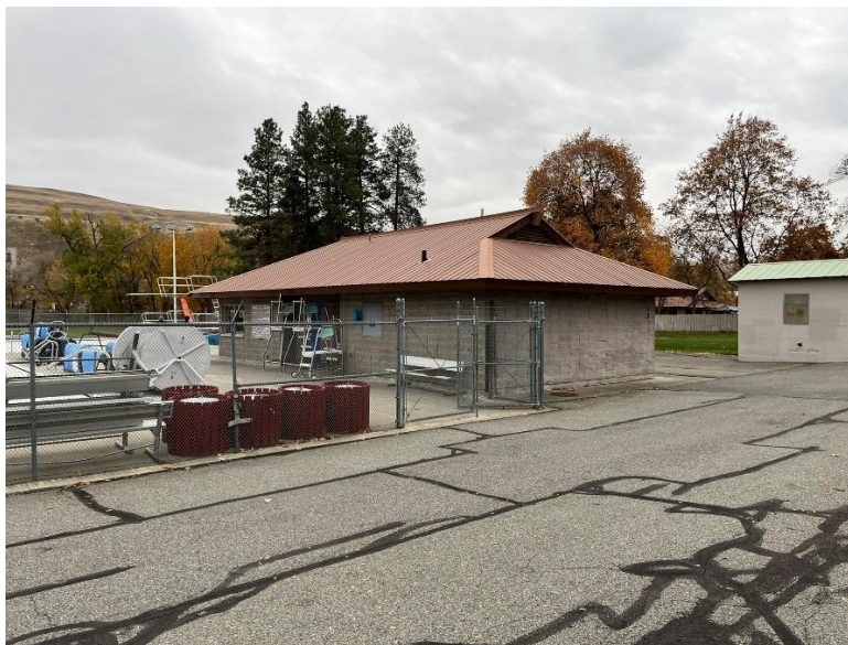
Plate 16 – Asphalt Cracking
