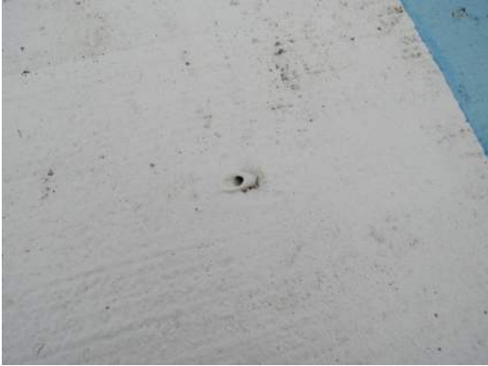
Stubbed floor return in pool floor
