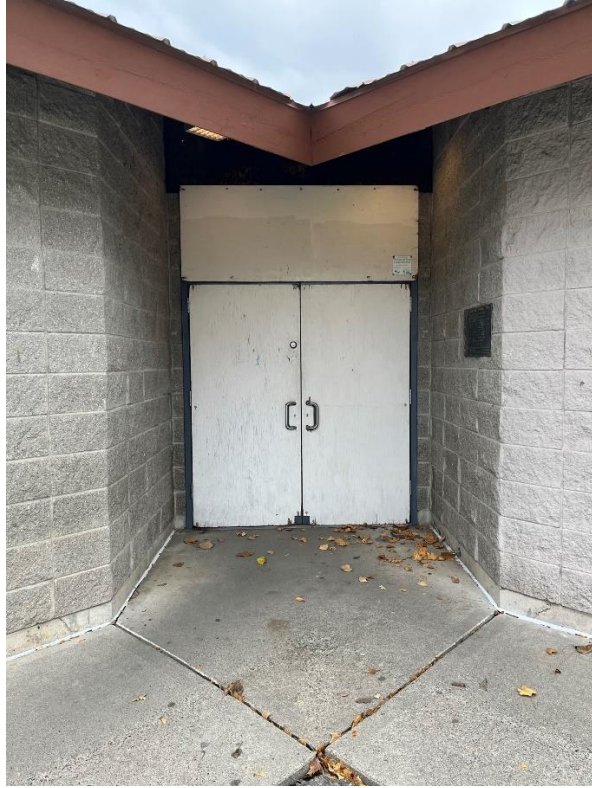
Plate 3 – Front Entrance Boarded Doors and Relite
