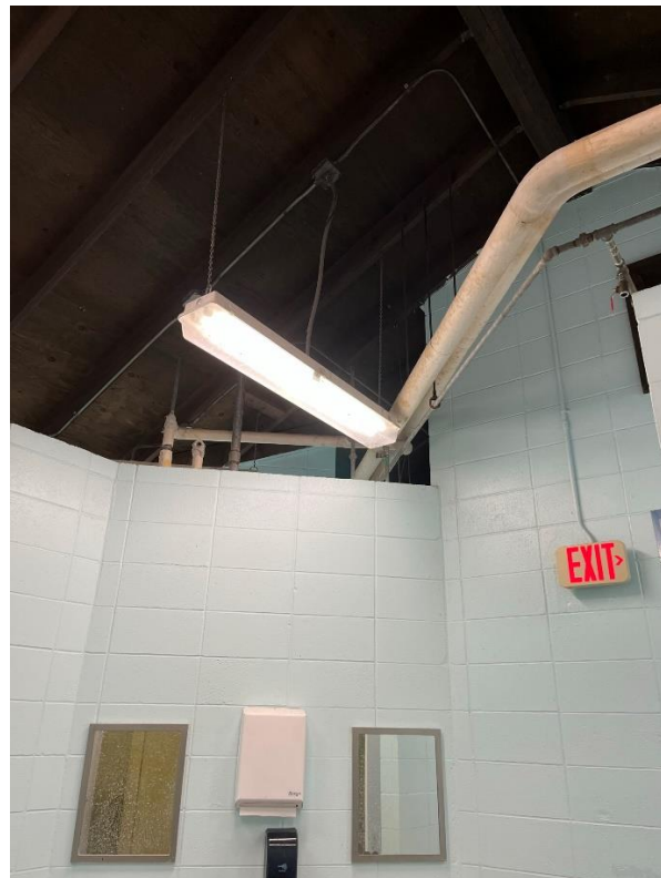
Plate 6 – Interior CMU Walls & Wood Framing
