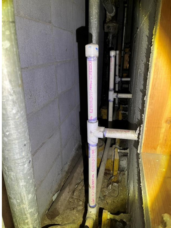
Plate 13 – Men's Restroom Wall Chase
